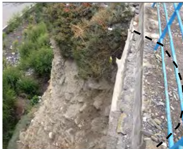
Recent failure near hotel, track undermined (not Annapurna Circuit) Track undermined, no support at edge
