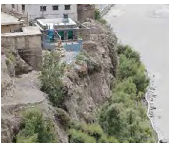
Recent failure near hotel, track undermined (not Annapurna Circuit) Track undermined, no support at edge
